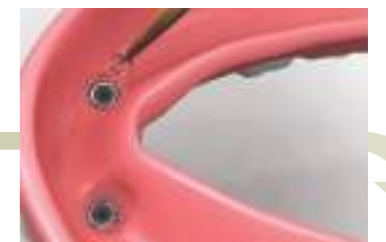
Apply resin around the female sockets.
